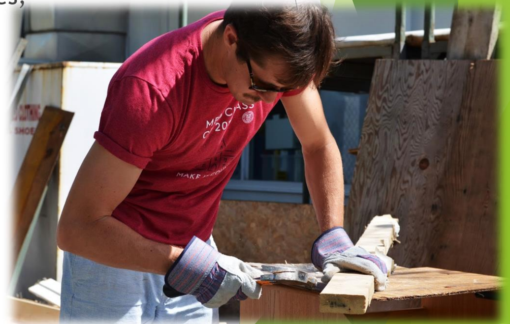
ReUse volunteer denailing deconstructed lumber
